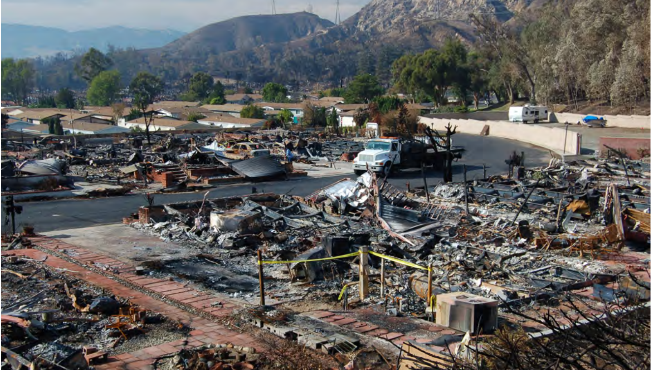
A Los Angeles mobile home park sustained heavy damage during a 2008 wildfire. Continued development in the WUI results in heightened risks for homeowners and businesses (Image Source: Wikimedia)
